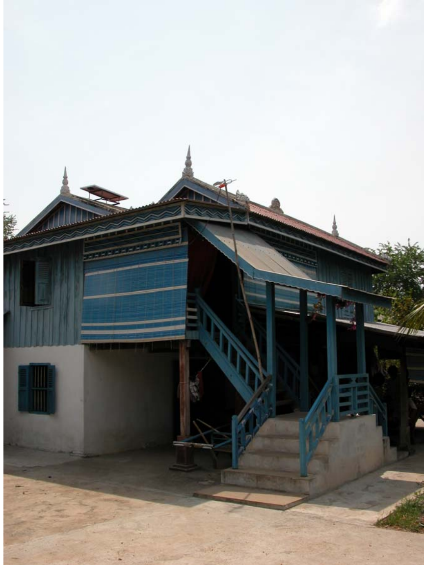
Figure 2: Cambodian Home with Solar Panel on Roof (author photo)
